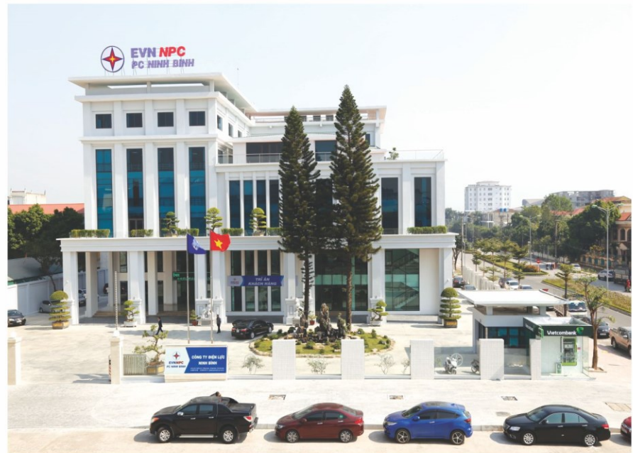
Headquarters of Ninh Binh Power One Member Co., Ltd
